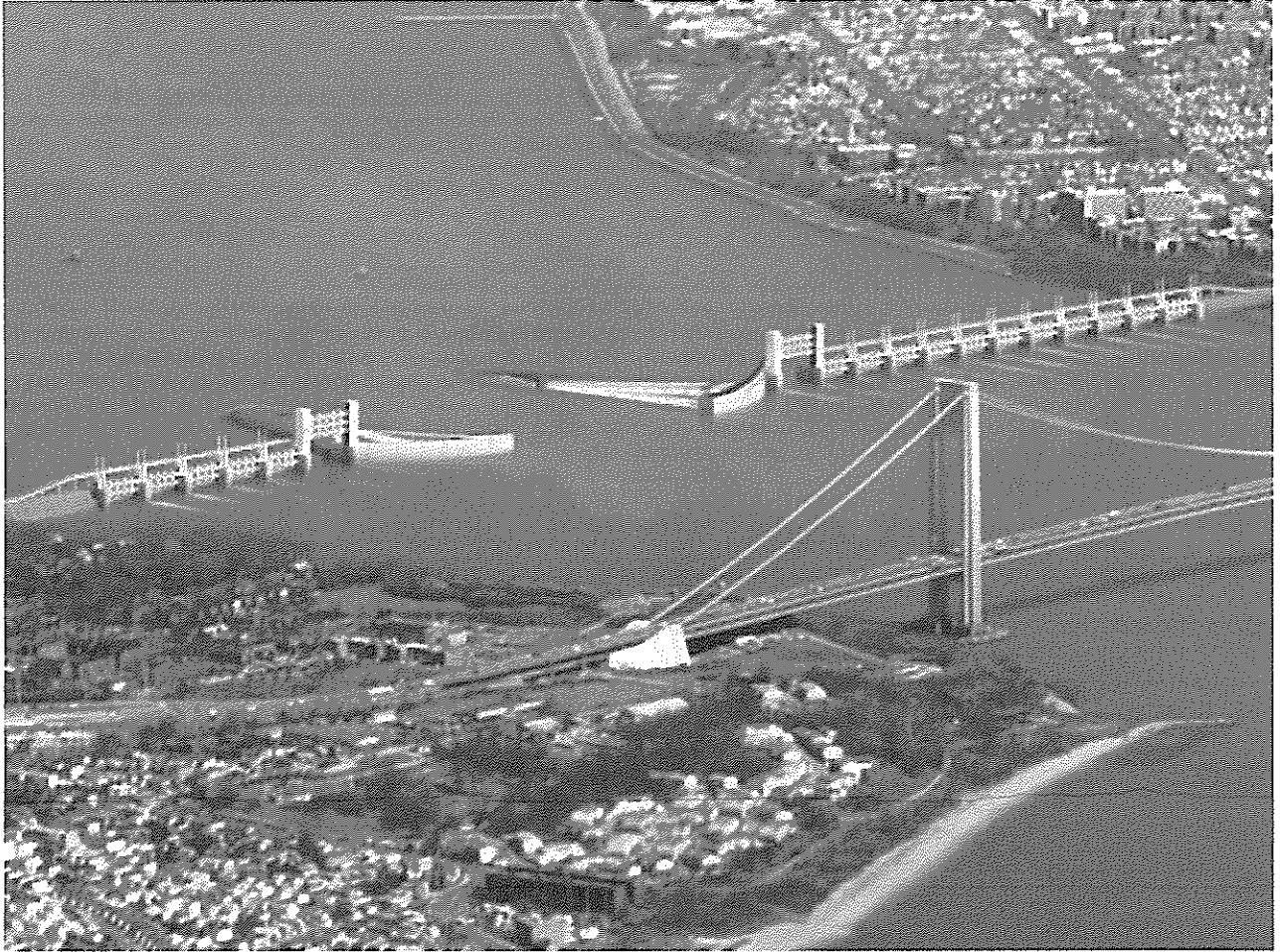
Figure 3. Proposed hurricane storm surge barrier for New York City near the Verrazano Narrows Bridge. Image credit: Arcadis, Inc.
