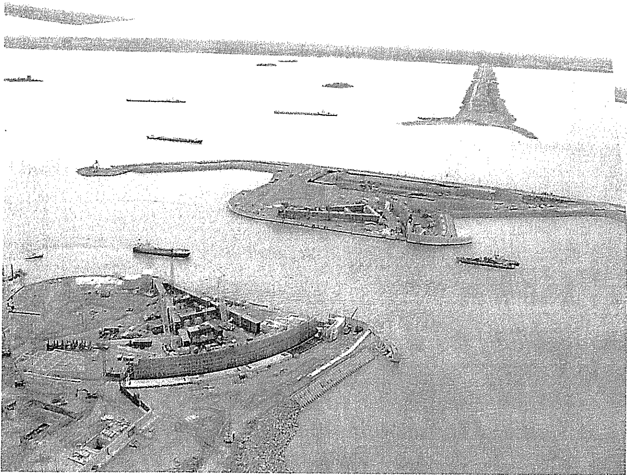
Fig. 3: Ring road and storm surge barriers presently being constructed around St Petersburg, Russia.
