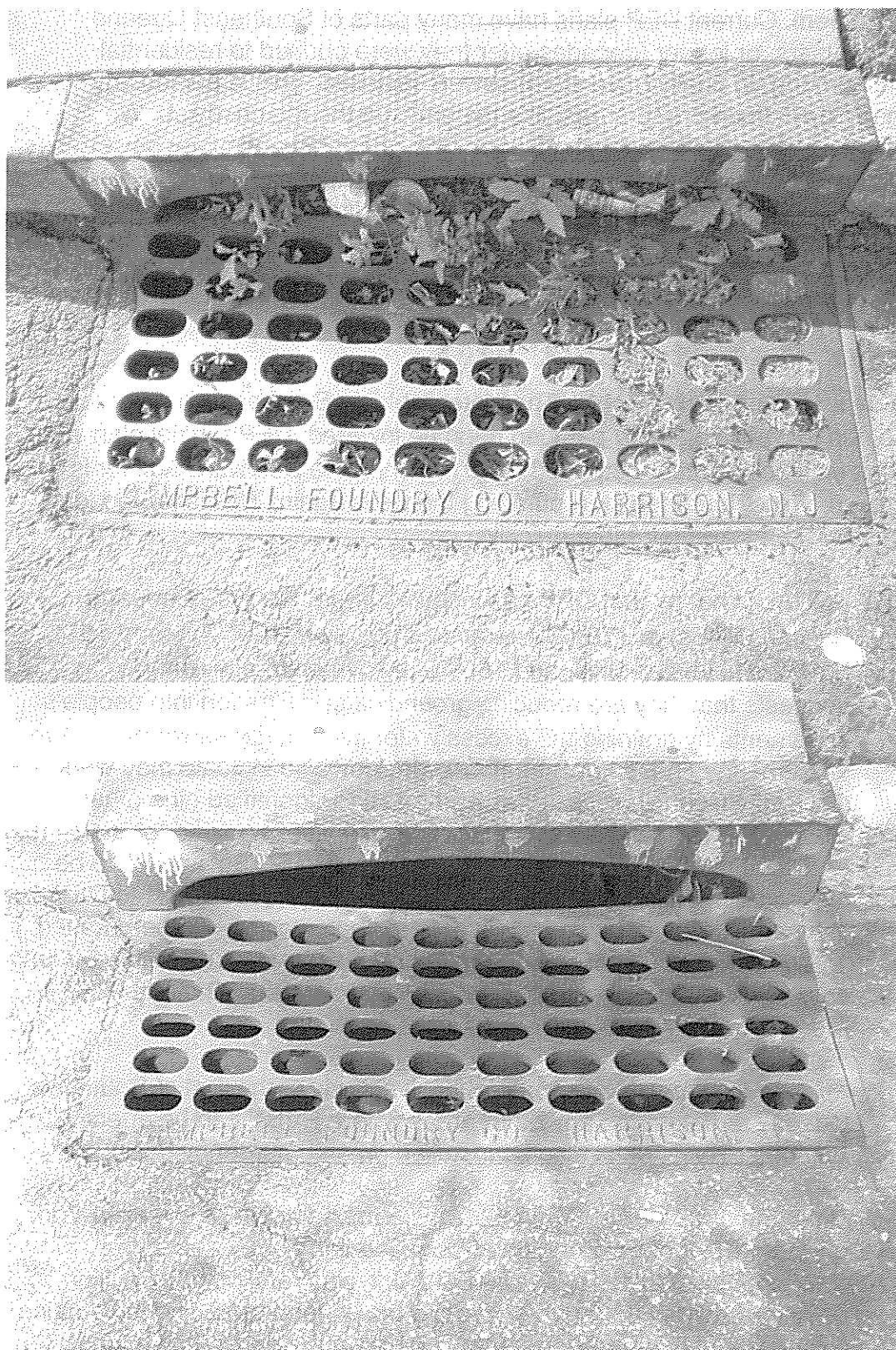
Catch Basin on Baisley Blvd, near Smith Street before and after cleaning
